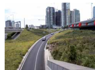
ABOVE: The Power Street on-ramp
